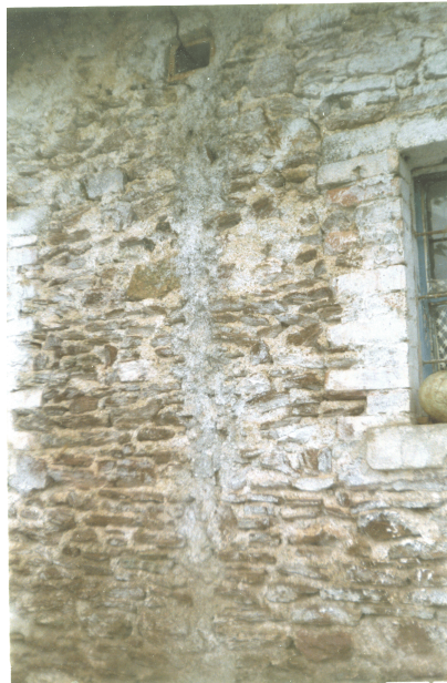
Cracks of the village houses walls
