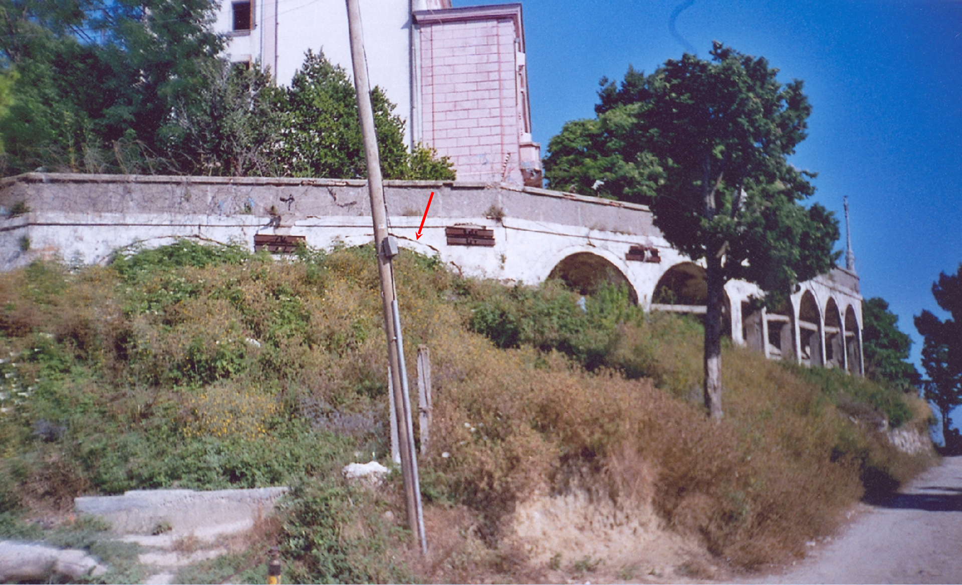
CRACKS OF THE KING ZOGU VILLA WALLS
