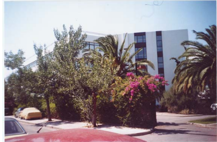
Photo 3. THENAMARIS Ships Management Inc. building, Athens, Greece where is successfully worked Borehole-Heat Exchanger-Geothermal Heat pump System for space heating and cooling
