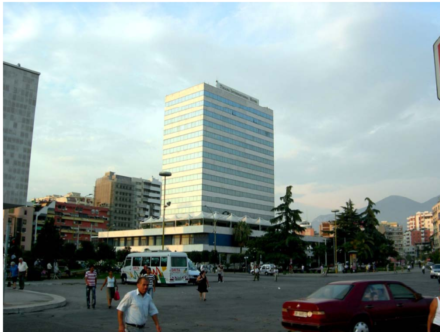
Tirana International Hotel Climatization by air-air chillers.
