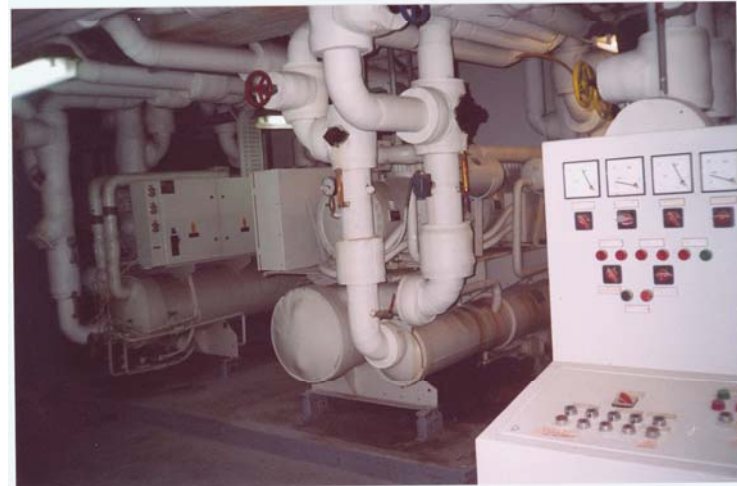
Photo. 4. Geothermal Heat Pumps installed in the THENAMARIS building
