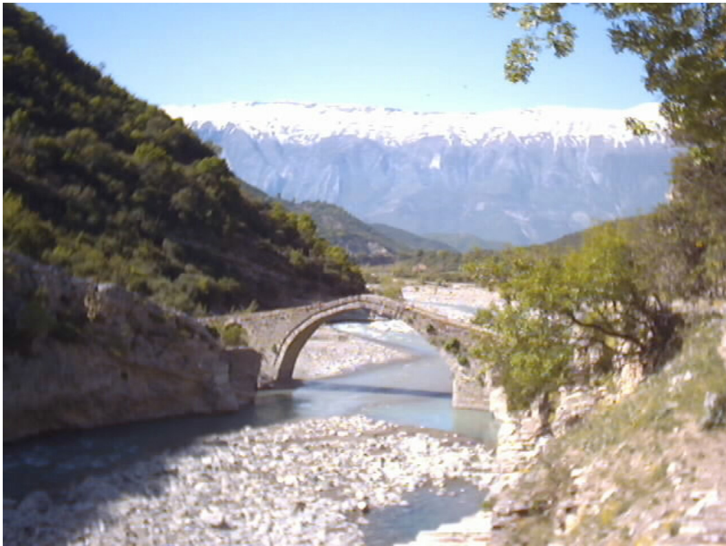
Photo 1. Langarica-Permeti thermal water springs
