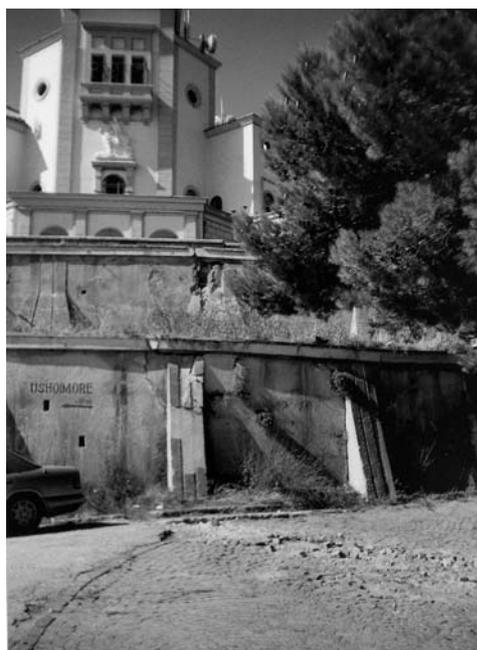
Photo 3.12. Cracks in the villa walls and transversality of the road
